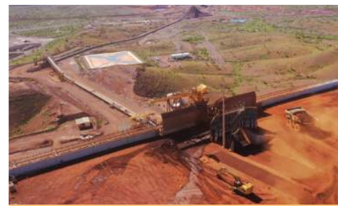
Gudai Darri ROM Containers
